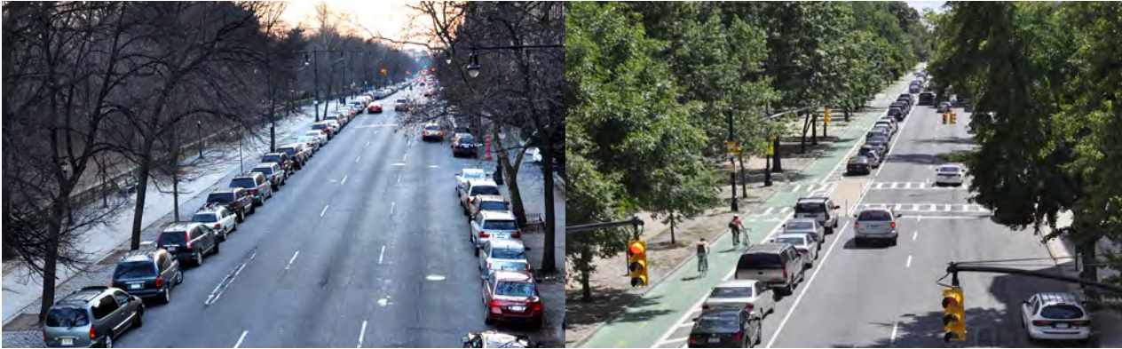
The insertion of a cycle track on this Brooklyn street dramatically improved safety for all road users without reducing daily car through-put
